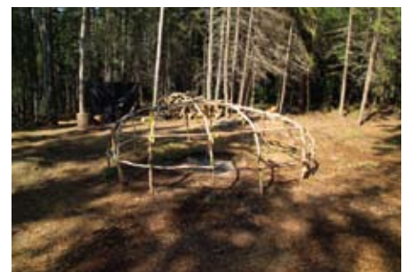
Construction of a sweat lodge near Wuskwatim Lake.
