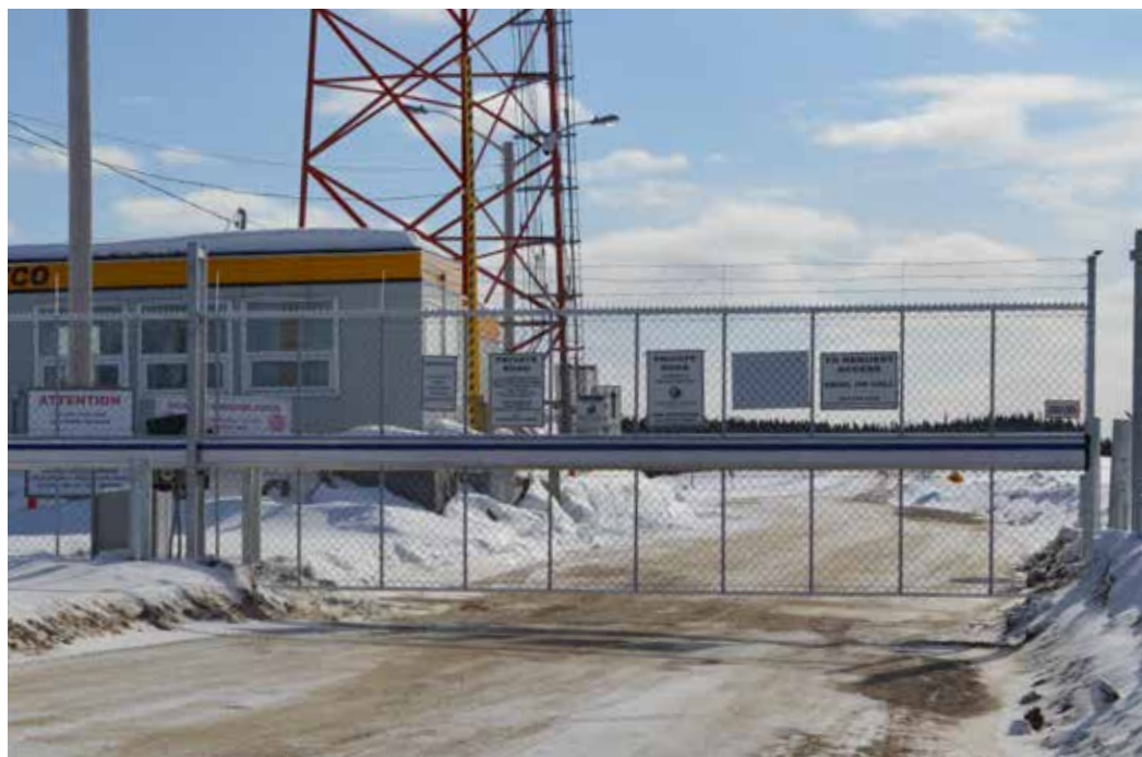
A fully automated gate was operational by late February 2014.
