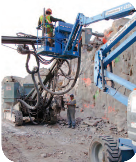
Rock bolt drilling operation on rock face.
