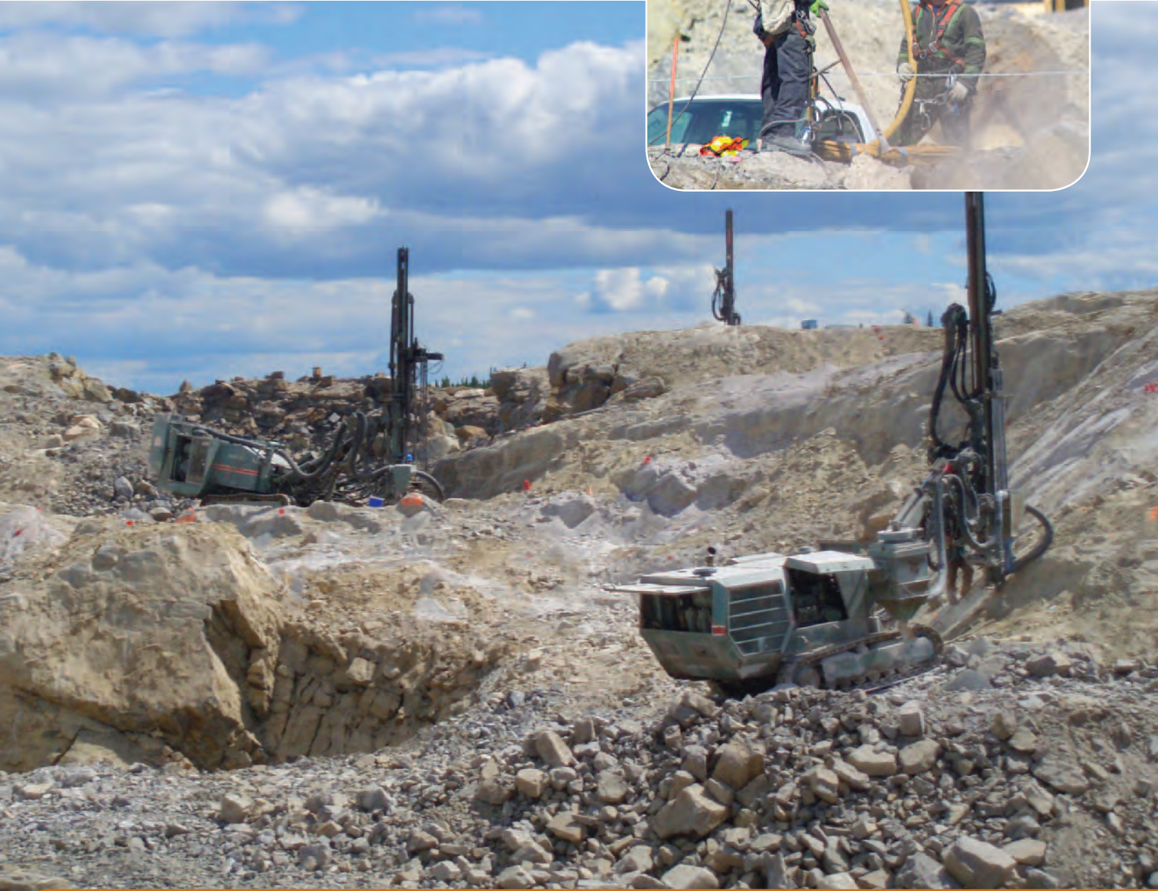
Rock drilling operations in preparation for blasting in the excavation area.
