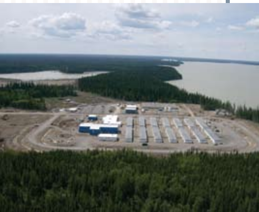
Construction camp near Wuskwatim Lake.
