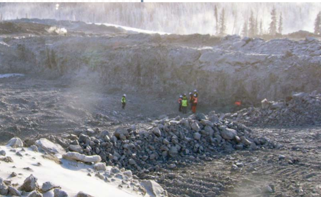
Inspection of excavation at spillway channel.
