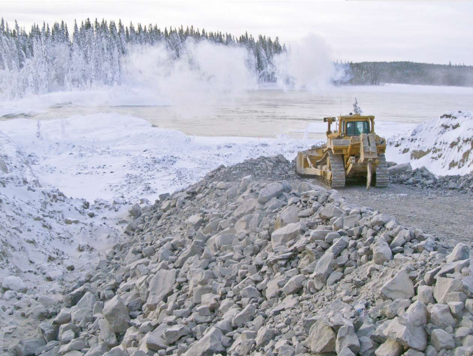
Constructing the ramp to begin the construction of upstream cofferdams.
