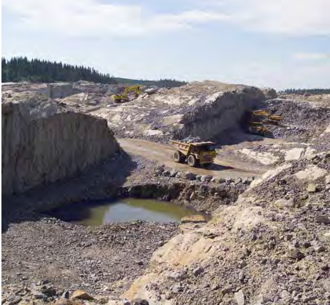
Excavation of the spillway channel.
