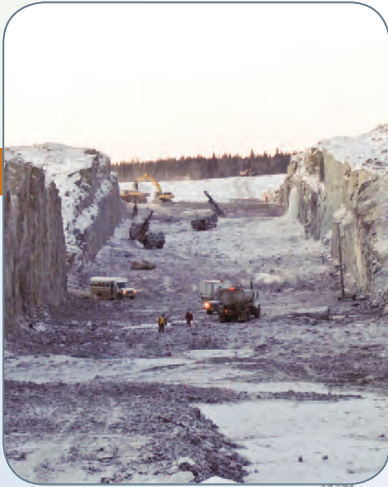
Rock excavation activities in the spillway channel.
