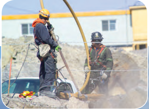
Workers using compressed air to remove loose rock and debris in excavation area.
