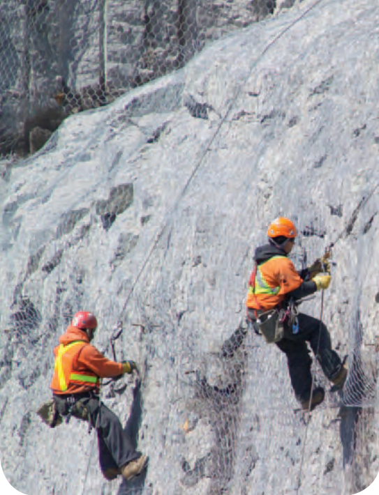
Construction workers suspended on rock face in spillway channel attach wire netting to secure loose rock.
